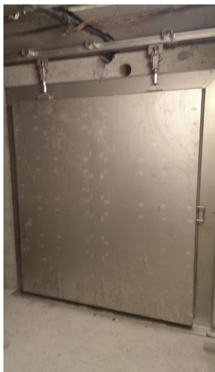
This sliding watertight pressure door (1.7 x 1.9 m) protects the equipment room at the Mapragg reservoir in Bad Ragaz CH, which otherwise could be inundated in case of an extreme flood event.
