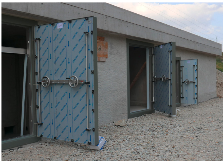
Watertight pressure doors protect the Füreli power plant against avalanches in Hinterrhein/CH
