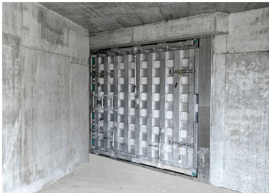
This watertight pressure door in the Lyssbach spillway gallery provides access for maintenance vehicles.
