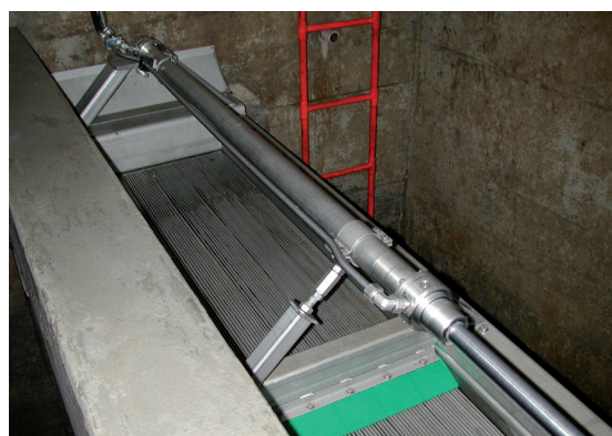
ROMAG CSO screen RSU. Relief end with hydraulic cylinder and cleaning carriage. Concrete sill forms the emergency relief.
