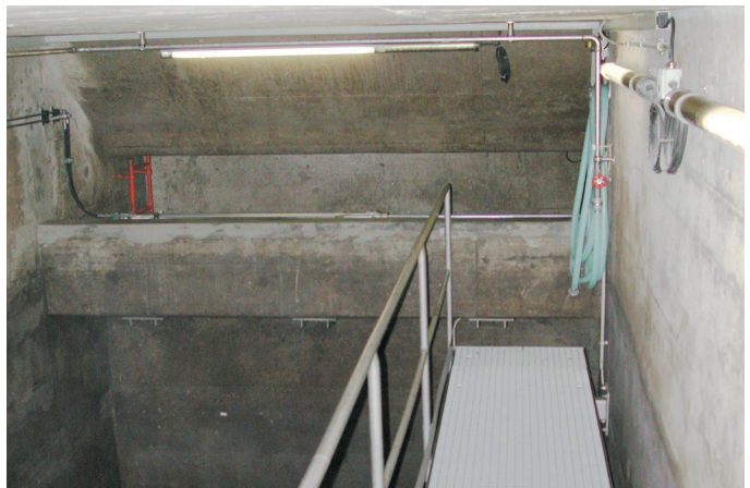
Zürich-Wollishofen sewage treatment plant, left basin half, ROMAG CSO screen RSU in the background. The hydraulic pipe for the cylinder is clearly visible. The hydraulic cylinder can just be seen above the edge of the masonry wall.
