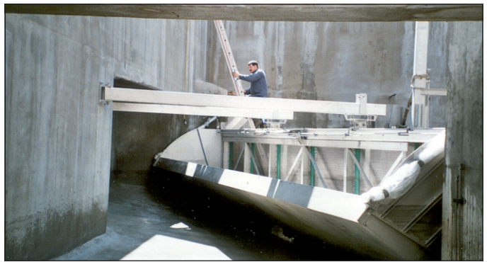
WWTP Telli at Aarau, ROMAG CSO screen RSW-K 14x8/4 (Built in phase)
