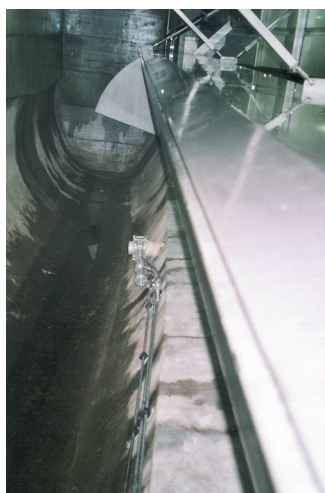
WWTP Kolben, RSW-K 11x8/4 Weir wicket closed
