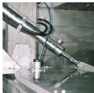
WWTP Kolben, Level probe
